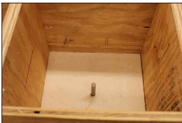
Figure 2-4: Photograph Showing at Typical Bottom Pin in Typical Formwork
