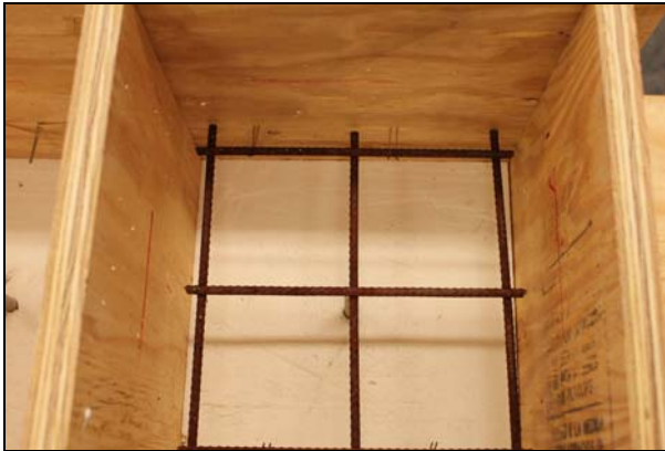
Figure 2-5: Welded Wire Reinforcement Placed Just above Bottom Pin
